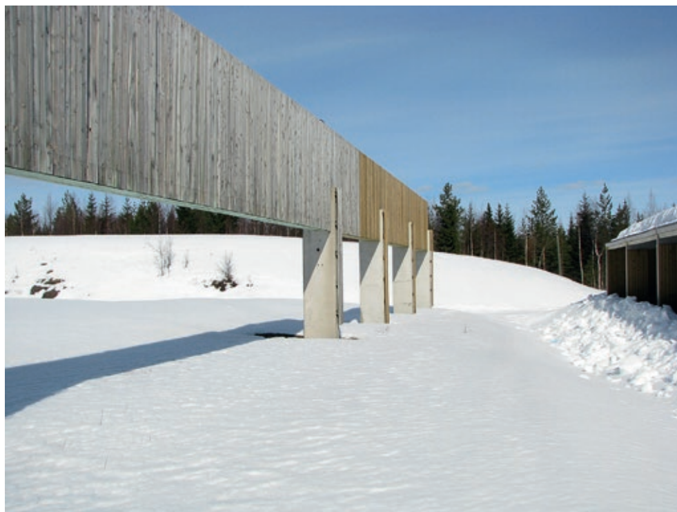
Figure 9.17. A baffle constructed to improve the safety at a shooting range.
