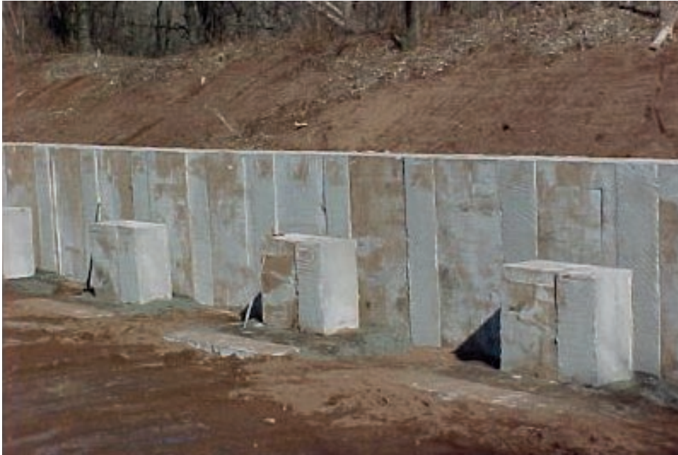
Figure 5.12. Sacon bullet trap during construction phase (Terran Corporation 2011).
