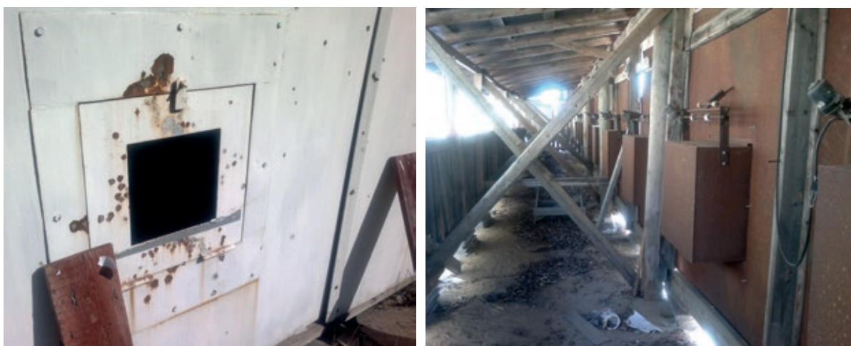
Figure 5.9. Jurva bullet trap from front and back.
