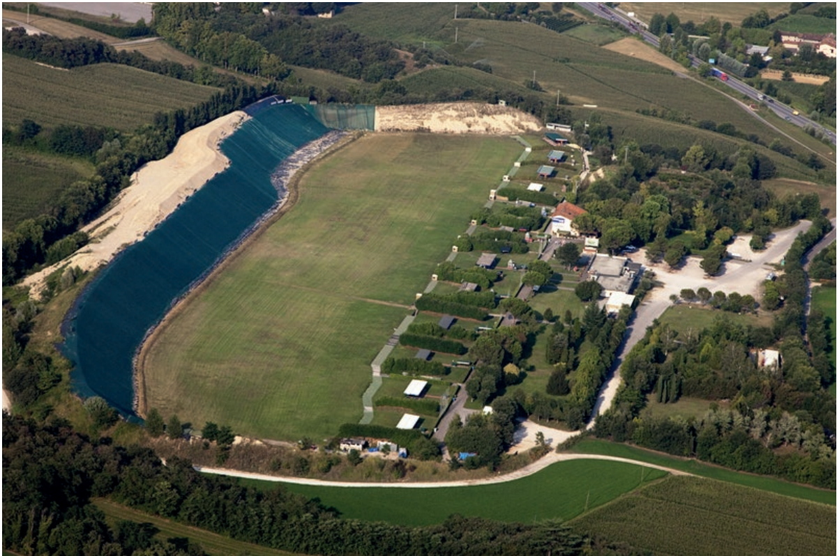
Figure 5.19. Berm structure at the Lonato shooting range in Italy (A.S. Trap Concaverde, Gallery).
