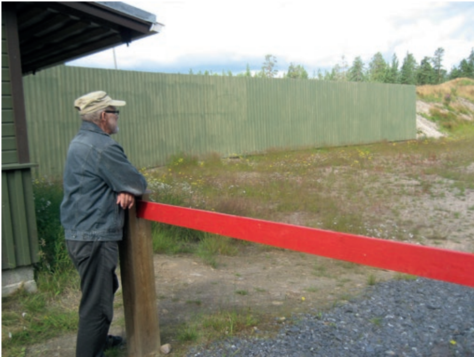
Figure 9.11. Sound-reflecting noise screen constructed at an elk target shooting range.
