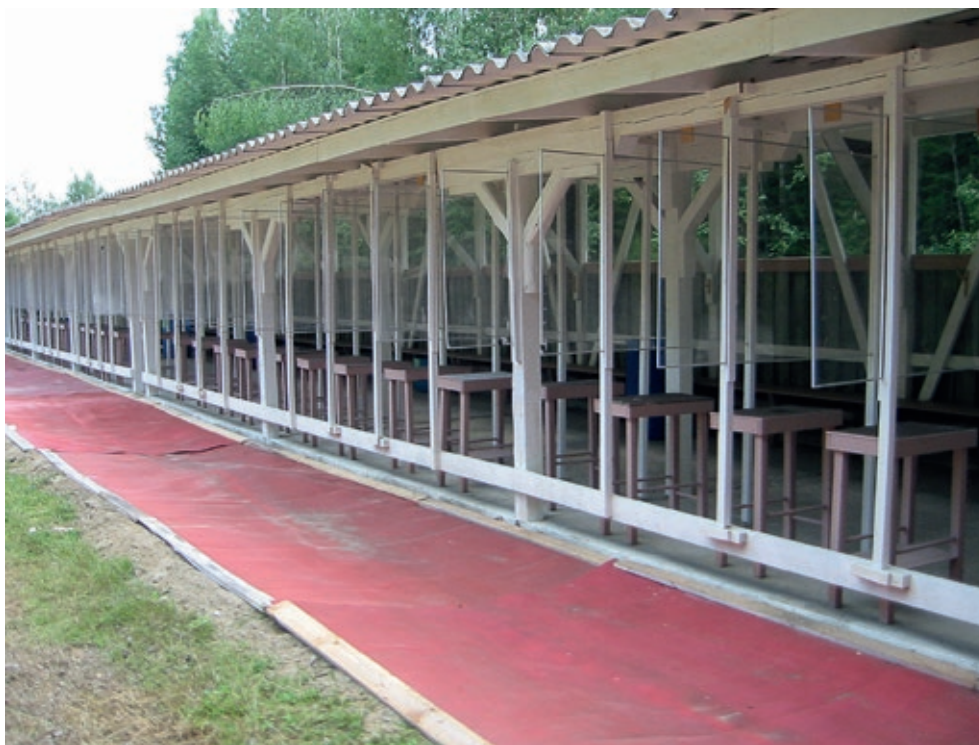
Figure A.2. Examples of a pistol range firing enclosure and its covered front (Keski-Suomen Ampujat, Laukaa). Photo: Jorma Riissanen
