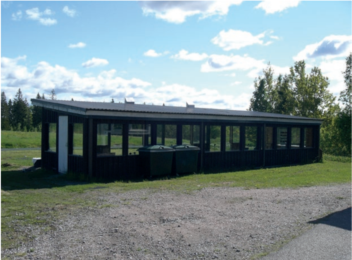
Figure 9.14. A trap shooting enclosure at the shooting range of Sipoon SSG, attenuating noise to the rear sector. The window openings have airtight glazing.
