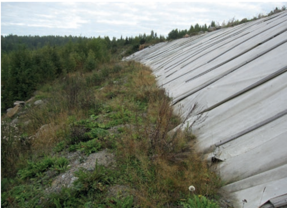
Figure 5.17. Backstop berm at the Nokia shotgun range (photo: Ramboll Finland Oy).
