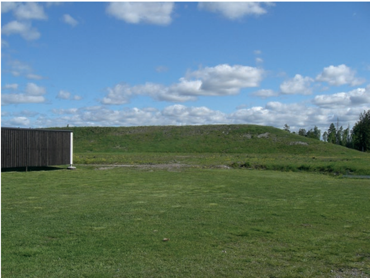
Figure 9.16. 15 metres high noise berm at the shotgun range of Sipoon SSG.
