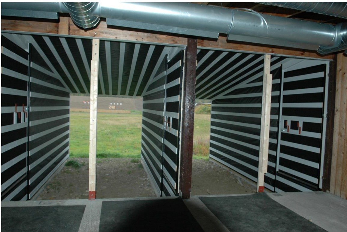
Picture 3.1. Semi-enclosed shooting range with noise cancelling. Picture from Råvatn shooting range.
